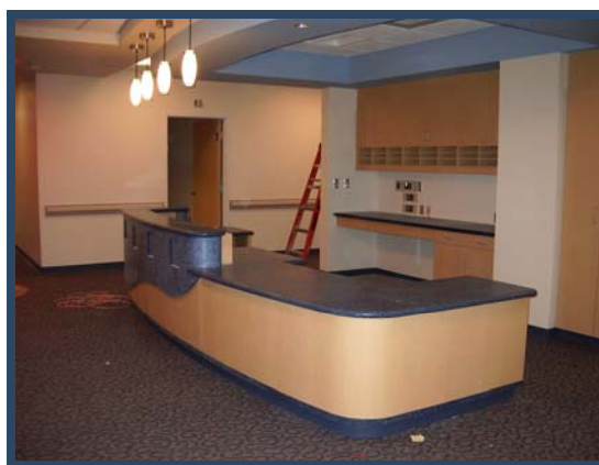
ACB under construction.
